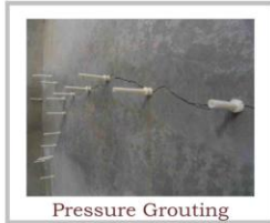
Pressure Grouting
